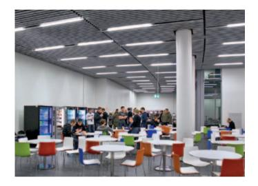
Most of the building has a specially designed ceiling system with perforated slat-shaped sheet metal segments which also integrates the illumination. Zumtobel won the competition for the best possible fulfilment of the diverse illumination requirements initiated by the client.
