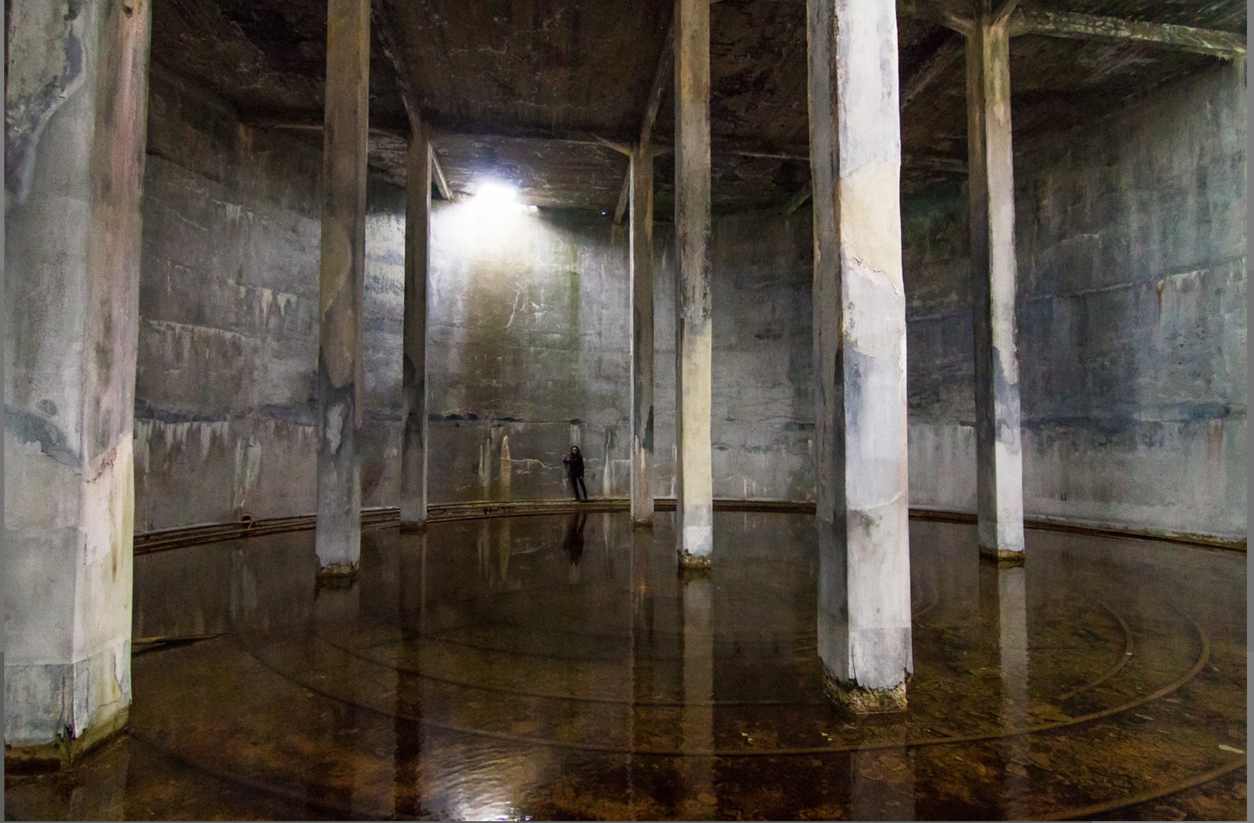
Fish-Oil-tank at Djúpavík
