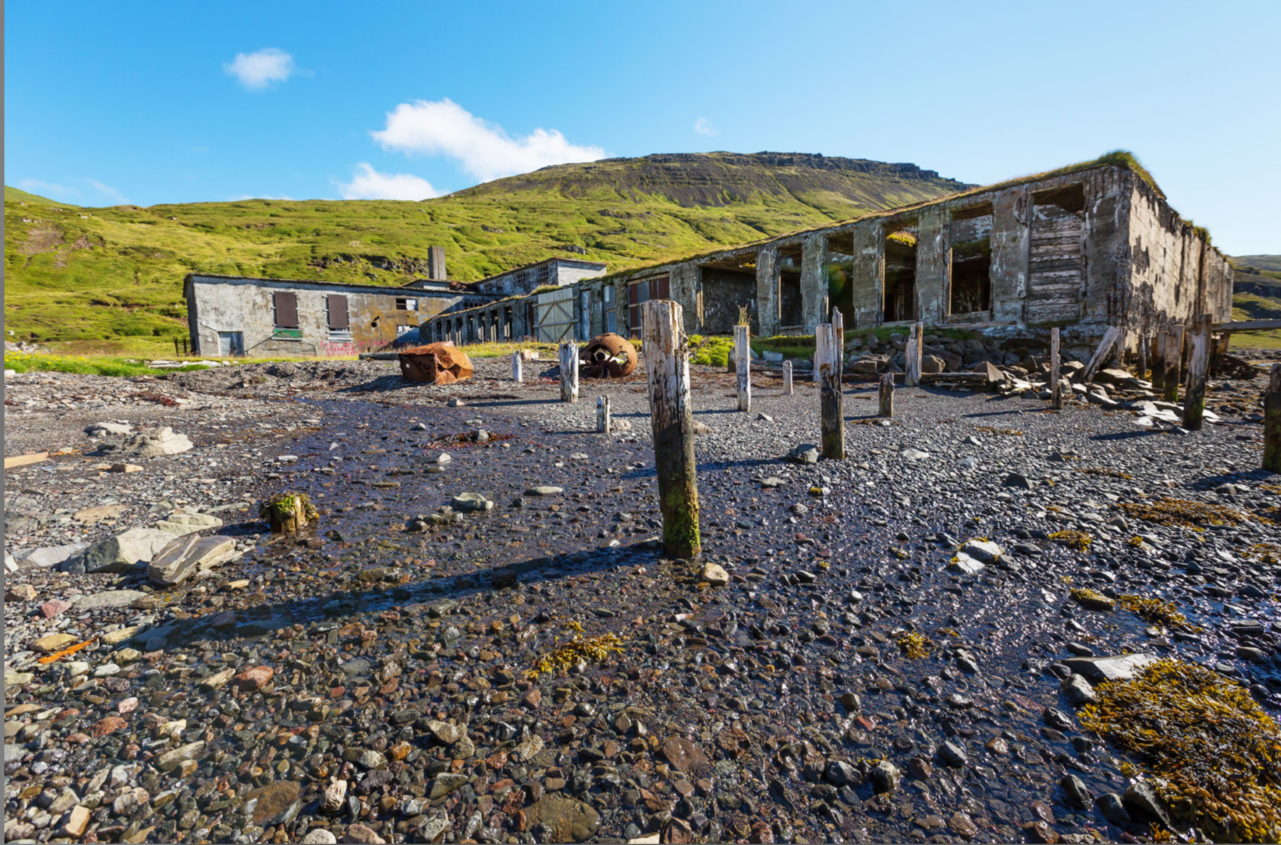
Abandoned Herring Factory at Eyri
