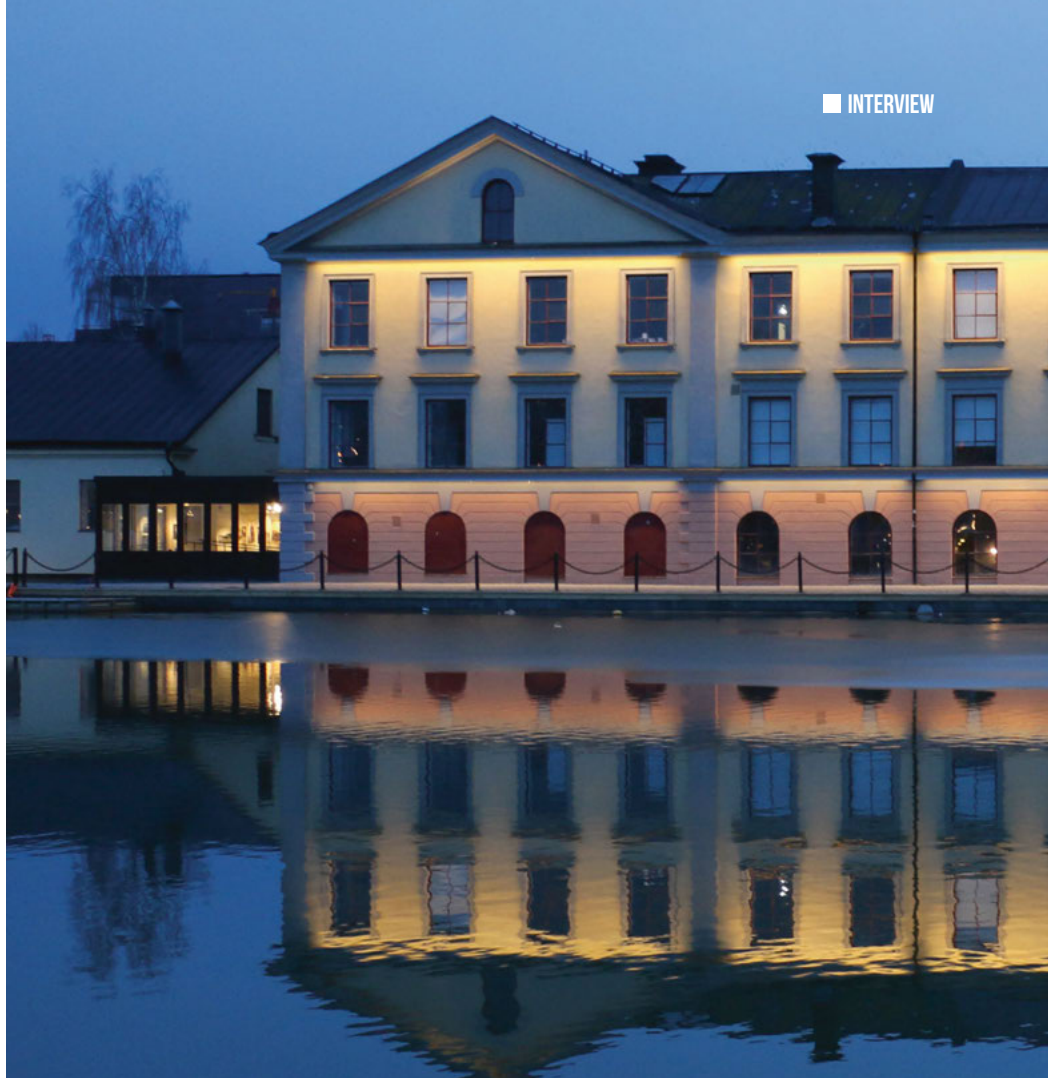
Left Because of its long periods of sunlight in Summer, and prolonged darkness in Winter, Scandinavians have a unique relationship with light. Above Eskilstuna City Museum, featuring lighting design from Tengbom, perfectly demonstrates the Scandinavian approach of 'lagom', of not too much and not too little.
