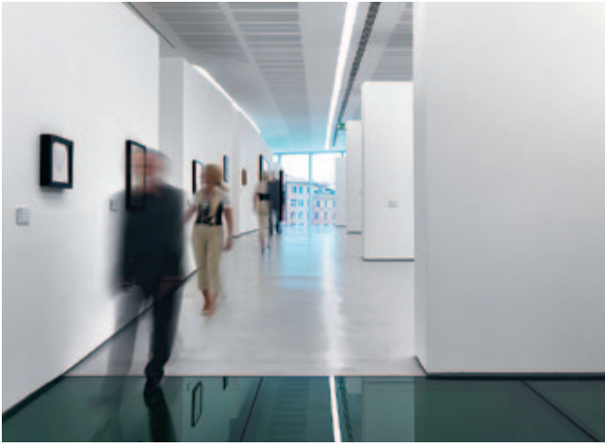
The lighting is integrated in the ceiling as a continuous light band and also provides an even illumination of the walls (top and right).
