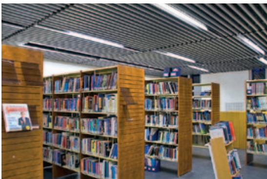
The illuminant specially developed for the building offers a very high efficiency despite its very small dimensions and fulfilment of the anti-glare specifications. The illuminant used is a visible, innovative T5 lamp.
